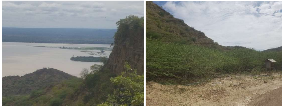
Left = Cliff with debris at the bottom (Facing- 70^\circ ), Right = Old Landslide (Facing- 50^\circ ),
